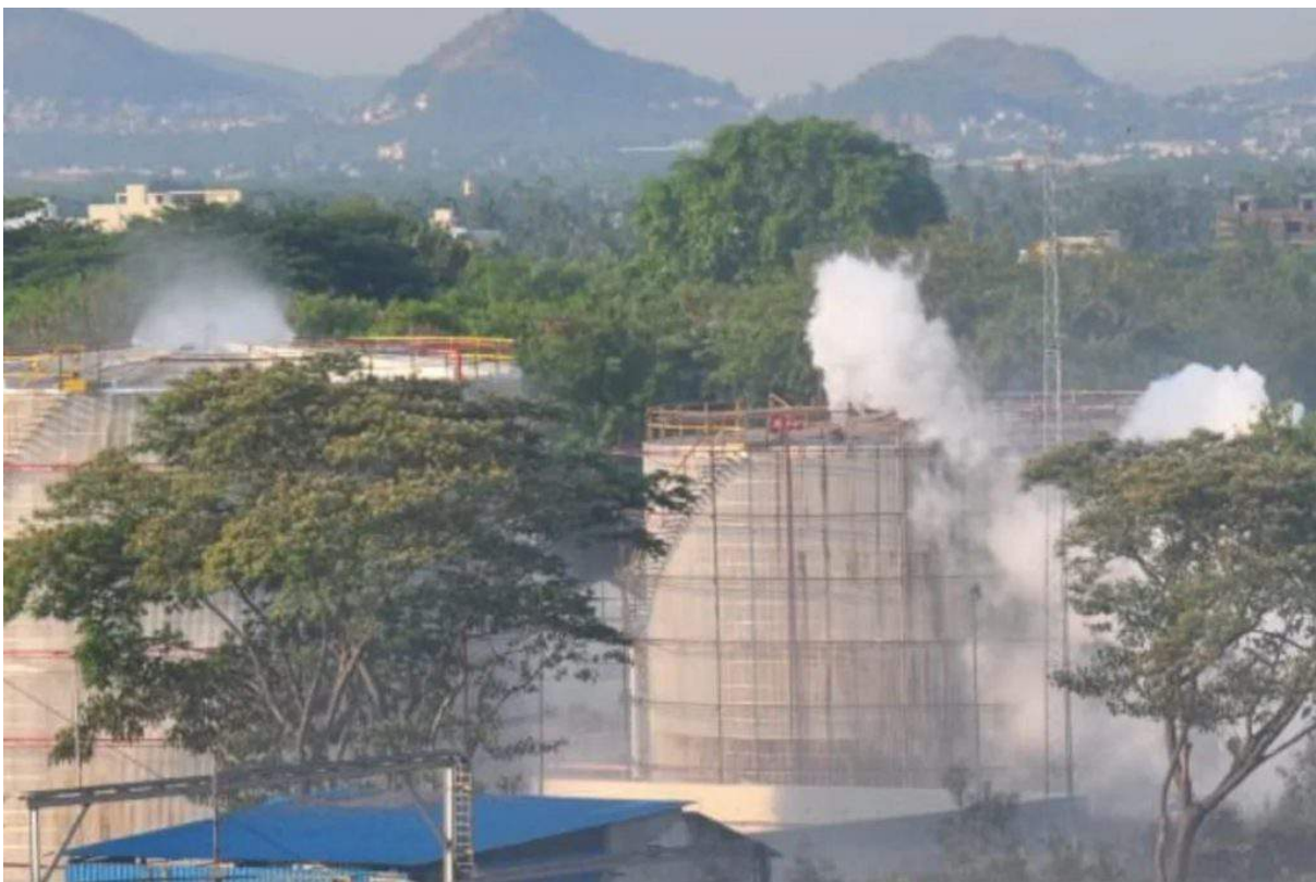
The May 2020 Vizag Gas Leak occurred as a consequence of a series of regulatory and operational failures, all of which could have been avoided if there were transparent and publicly accountable environmental regulation of the facility.
