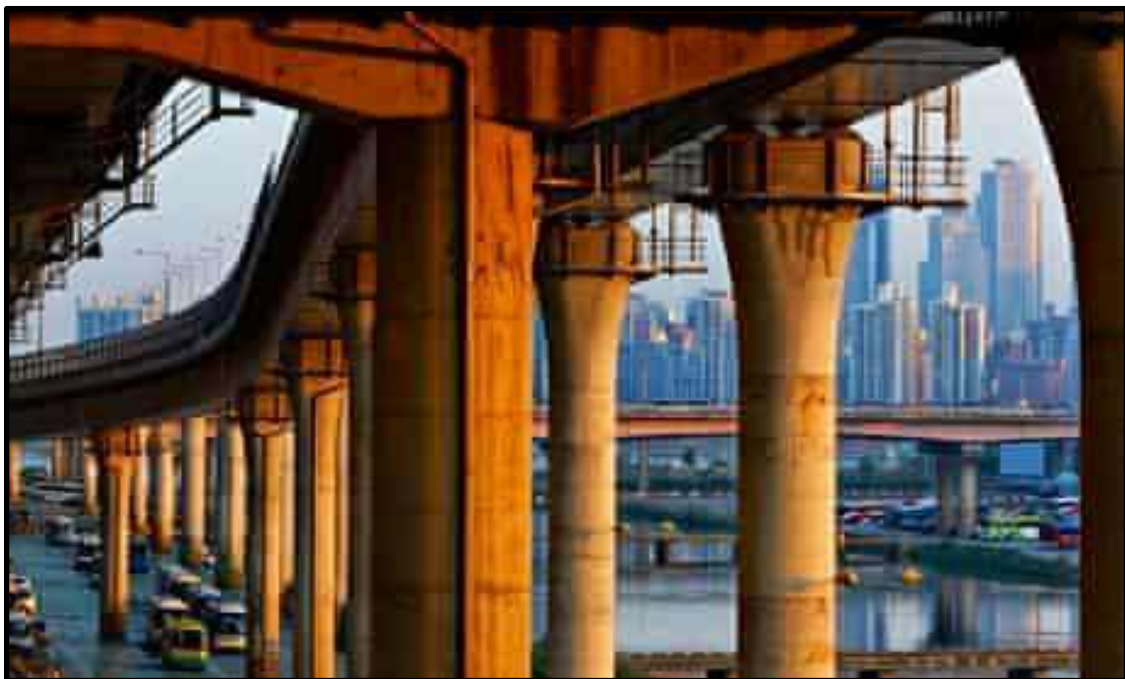
In 2014, Seoul's Ahyeon overpass was demolished and replaced by a greener, bus-only lane. Source: The Guardian, 13th March 2014.
